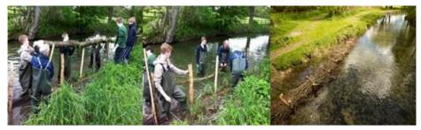
The team are narrowing the river by staking bundles of woody material parallel to the banks. The benefit of this is faster flow rates and the scouring out of silt, which is replaced by gravel in which trout lay their eggs. Faster flows should also encourage the growth of riverweed, which provides ideal habitat for the invertebrates which fish feed on.
