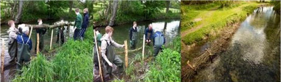
The team are narrowing the river by staking bundles of woody material parallel to the banks. The benefit of this is faster flow rates and the scouring out of silt, which is replaced by gravel in which trout lay their eggs. Faster flows should also encourage the growth of riverweed, which provides ideal habitat for the invertebrates which fish feed on.
