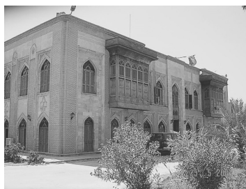
Figure (5): The building of the No. 3 British General Hospital as it appeared in 2003
